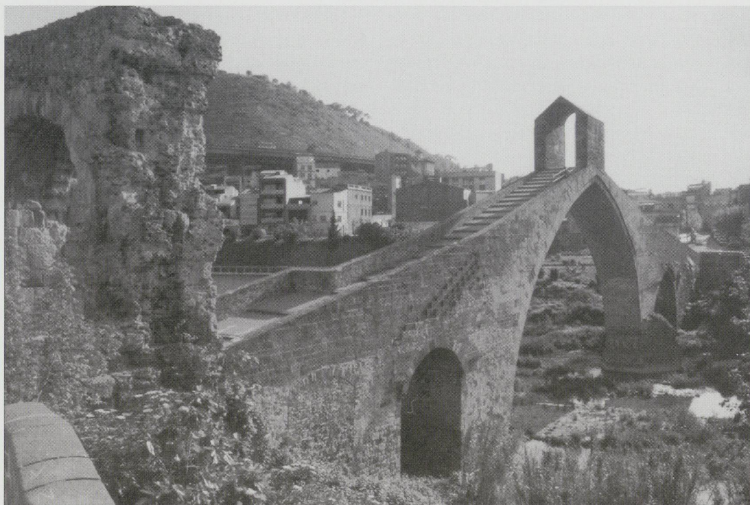
Fig. 3: Current overview of the bridge.
