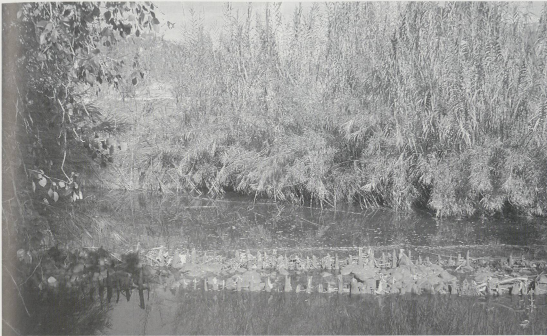
Fig. 2: Primitive dam system in the river bed of the Río Segura.
