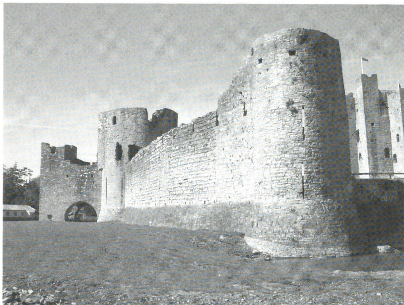
Fig. 3: Projecting from one of the towers on the curtain wall at Trim Castle, the barbican would have spanned the water-filled moat that originally surrounded castle.
