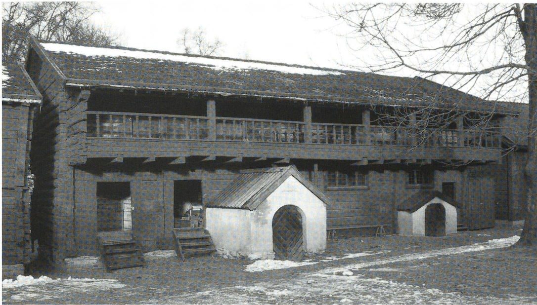
Fig. 3: Stone buildings are usually associated with high status, timber buildings with low status. But the medieval townscape included a significant, additional group – exclusive timber buildings – that scholars have largely ignored. The photograph shows a now-unique late medieval building in an urban environment – the Mayor's guest-house in Örebro, central Sweden (Photograph: Johan Anund).
