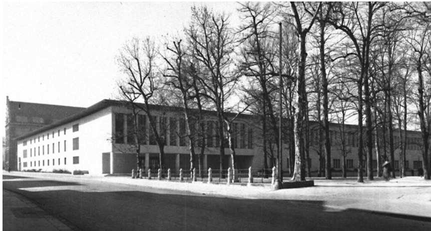
22 Main entrance with Petersgraben to the left and Petersplatz to the right, 1941.
